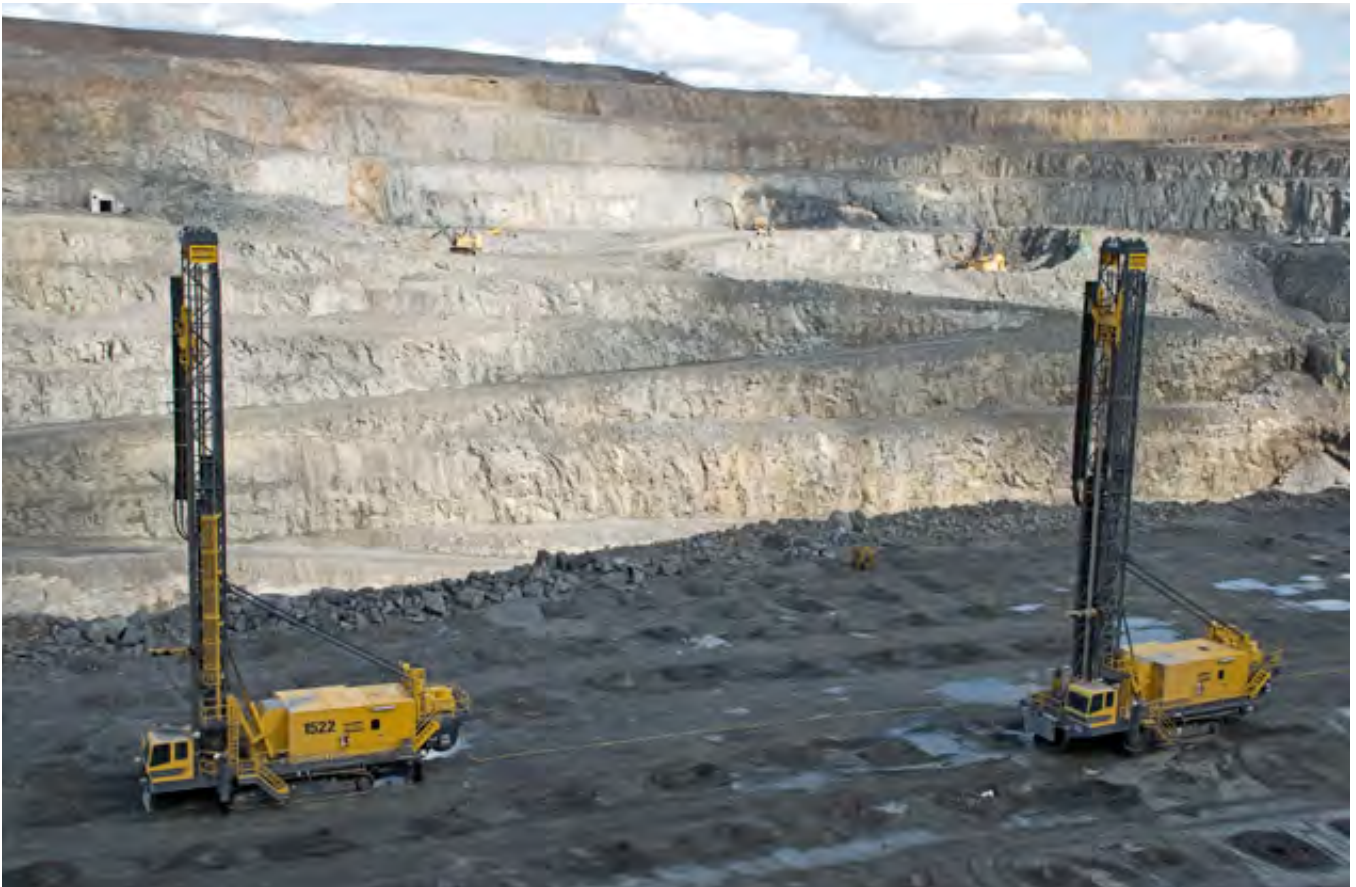
The drill rigs drill 200 – 300 holes for one blasting round and the penetration rate can vary between 0.4 m/min in the upper part and 0.1 m/min in the harder rock types. Orica is contracted to charge each hole with about a ton of Fortis Advantage emulsion. Drilling patterns are transmitted from the mine office to the Pit Vipers using the mine's W-LAN network.
