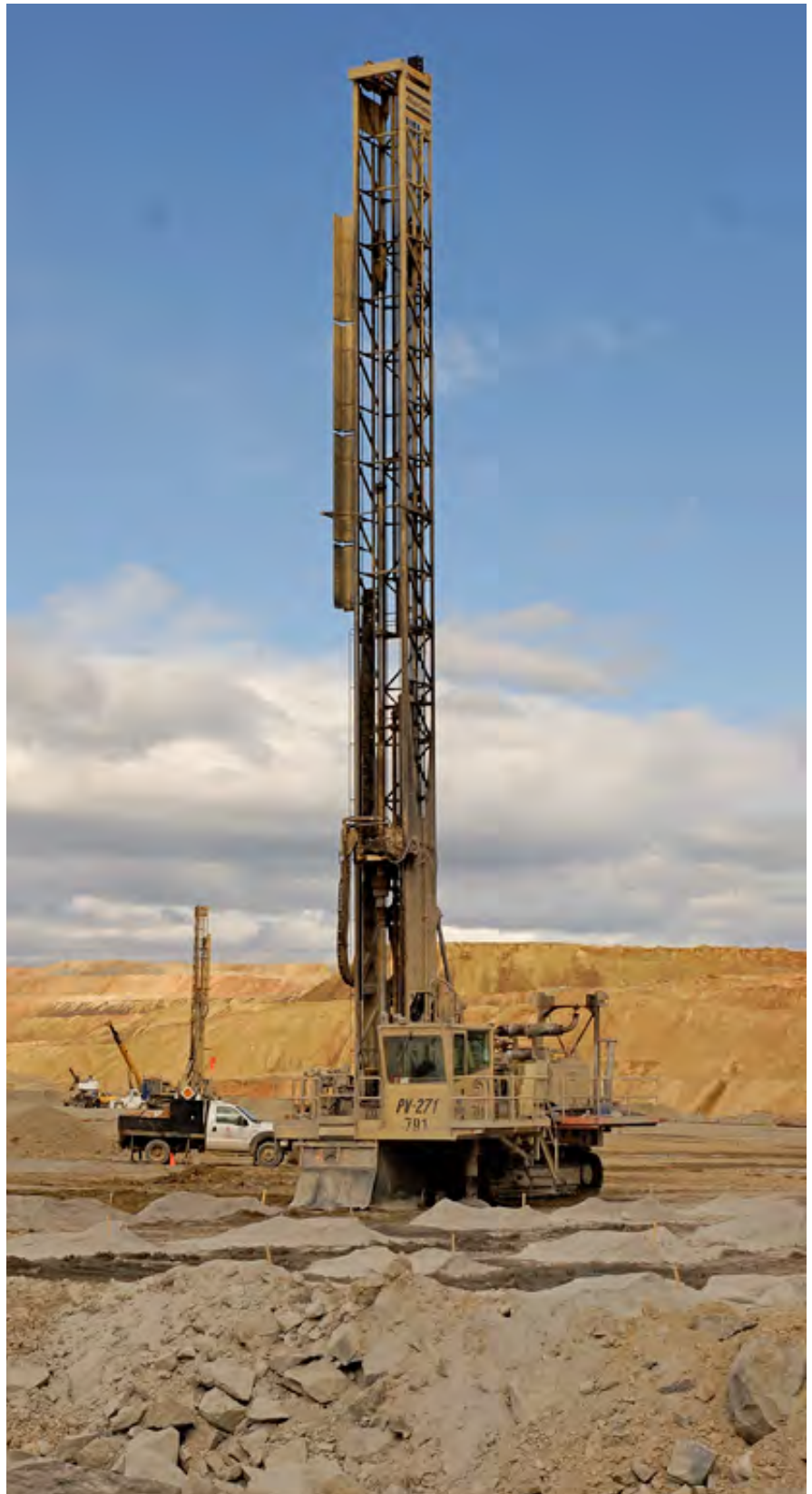
PV271's team up to quickly finish holes on a blast pattern.
